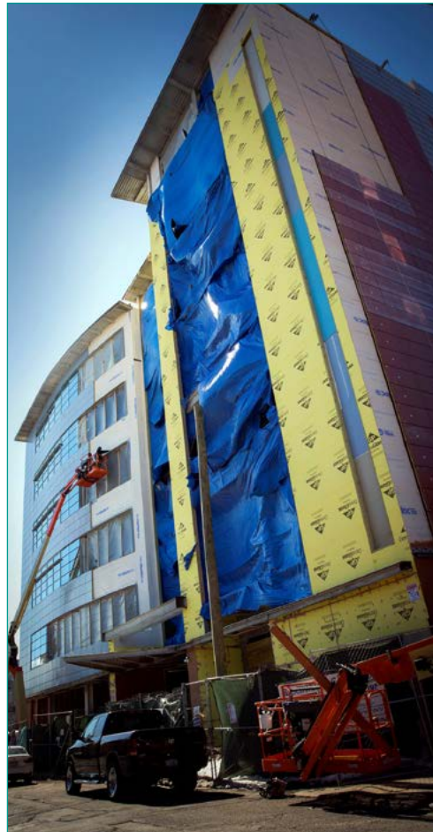
Exterior view of the STEM building currently under construction.
