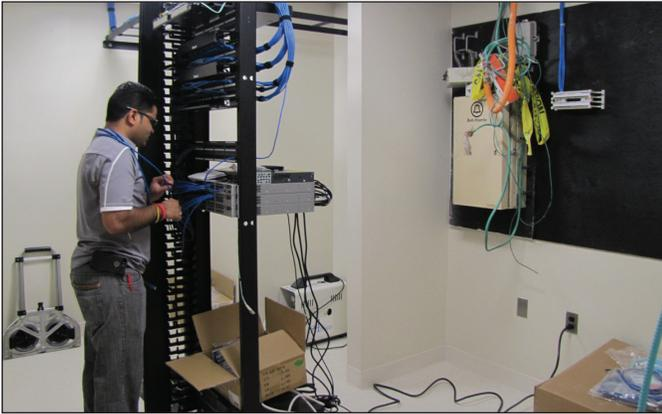
Hardik Sanghavi, PC Technician, patches a line on the Cisco switches, which connect the computers and printers to the College's server.
